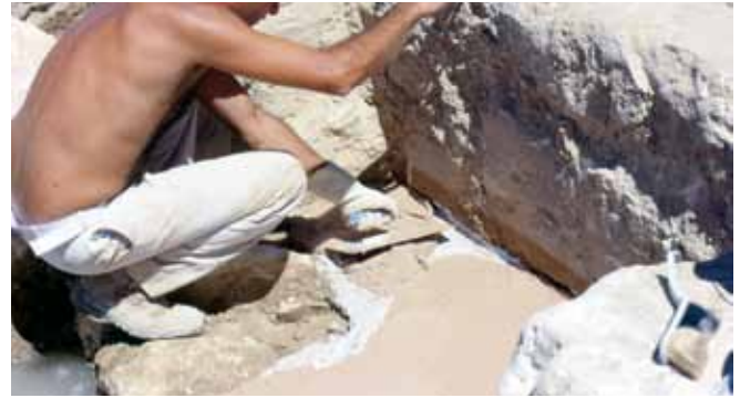
Figure 32. Lime-based hydraulic mortar is applied once the lime-wash undercoating has set.
