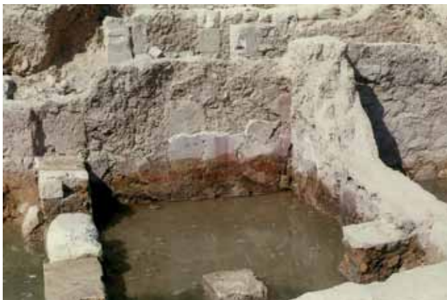
Figure 3. Area A being submerged without protective measures.
