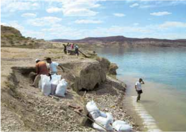
Figure 43. Positioning the bags filled with gravel.
