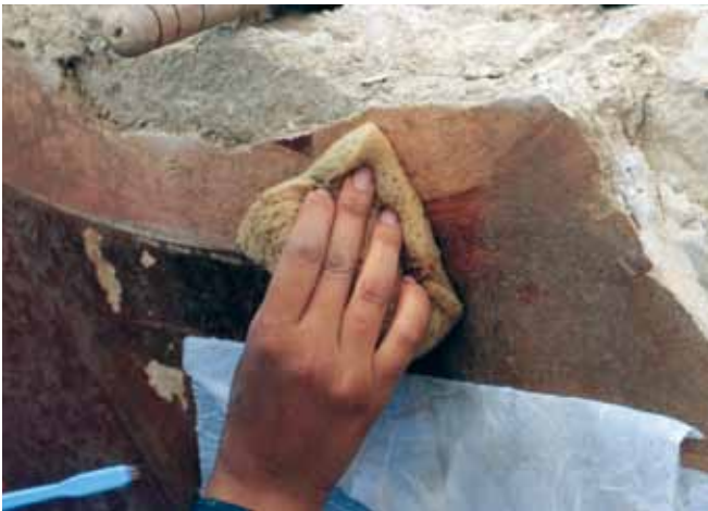
Figure 11. Cleaning performed with soft plastic brushes, synthetic sponges, and a 2 percent solution of NeoDesogen in water.
