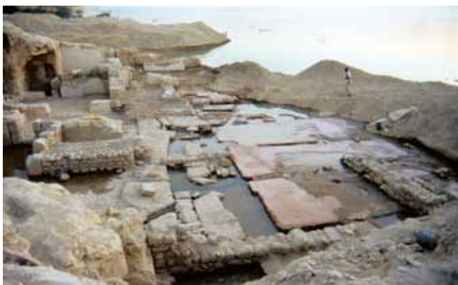
Figure 40. Trench 6, view to northwest, where reburial was not implemented and the structures were inundated with only hydraulic mortar for protection.
