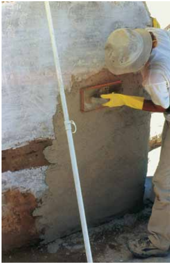
Figure 34. Lime-based hydraulic mortar is applied once the lime-wash undercoating has set.
