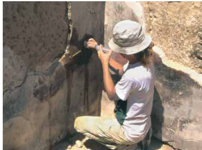
Figure 27. Deep grouting of painted plaster with hydraulic lime and brick powder.
