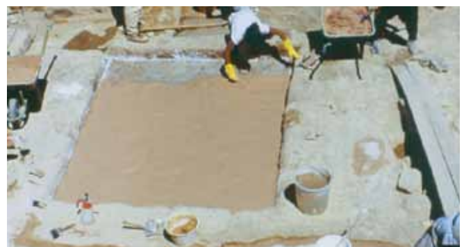
Figure 33. Lime-based hydraulic mortar is applied once the lime-wash undercoating has set.
