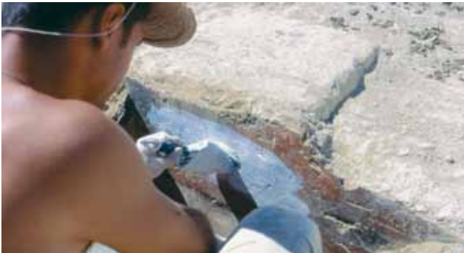
Figure 29. A layer of lime-wash applied to the surface of mosaics and painted plaster.
