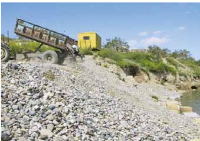
Figure 44. Filling in the terrain behind the bags with stones.
