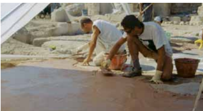
Figure 31. Lime-based hydraulic mortar is applied once the lime-wash undercoating has set.
