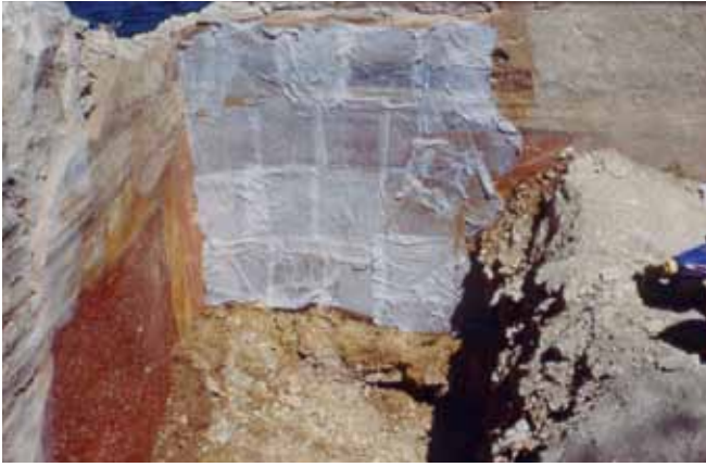
Figure 14. Wet tissue paper applied to painted plaster as a deterrent to damaging soluble salts.
